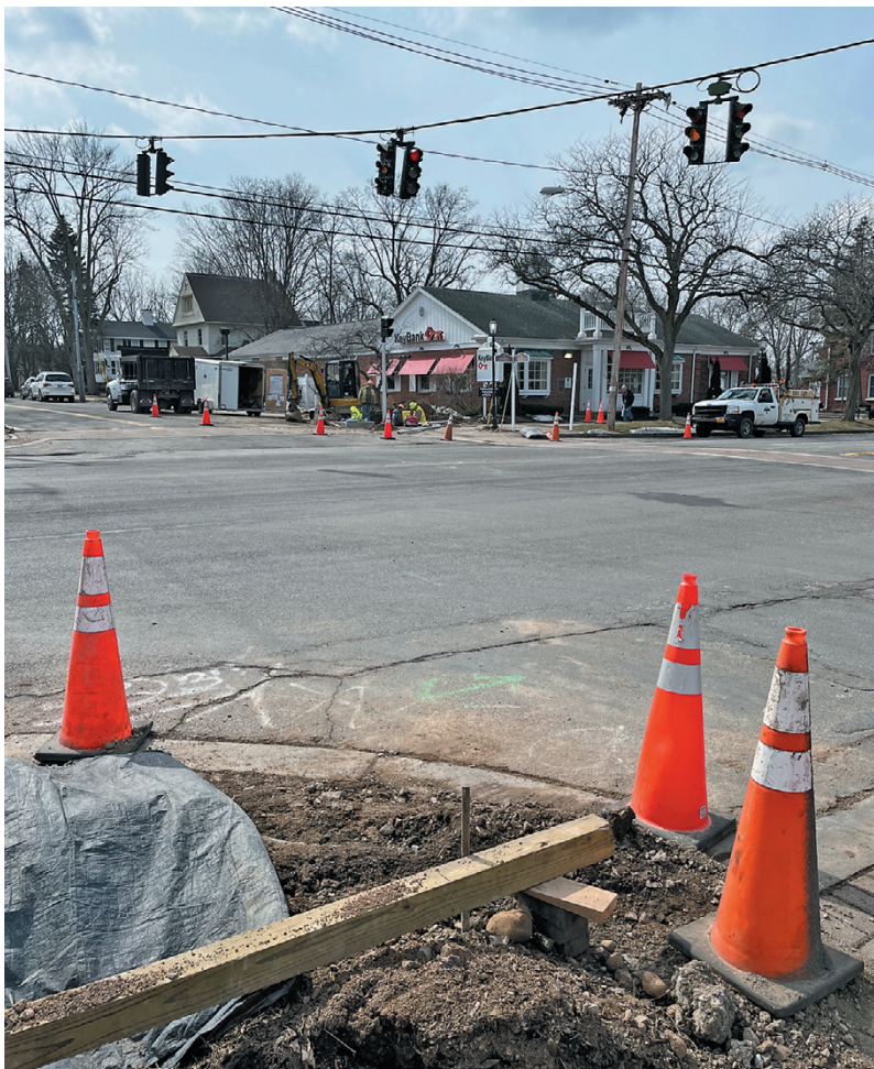
The Center Street face-lift process has commenced.
